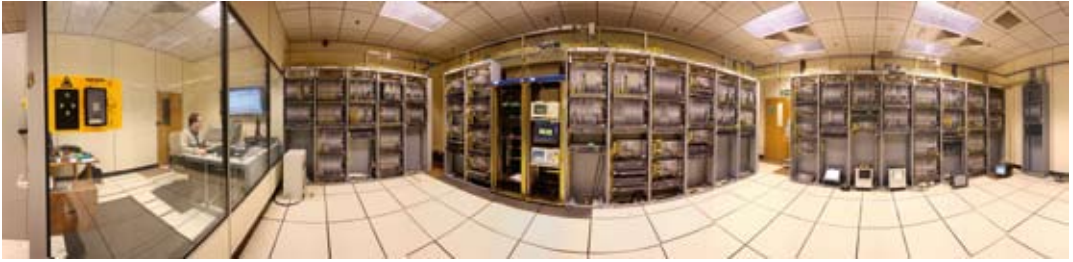
Fig. 4.1.17 System test environment © Ericsson
